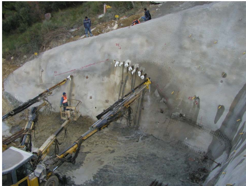
Figure 4. Pipe roof installation [3]
