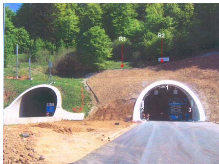
Figure 5. The Sleme Tunnel portal with marked positions of the right tube measuring points 1, 2, 3, R1 and R2
