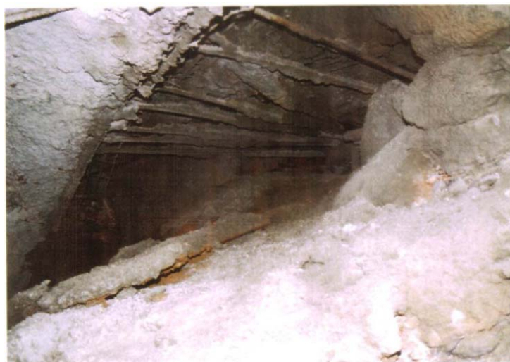
Figure 3. Excavation protection with piling [3]
